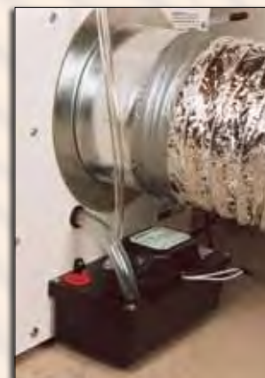
A SaniDry™ Basement Air System installed in the unfinished area, ducting dry filtered air into a finished area.
